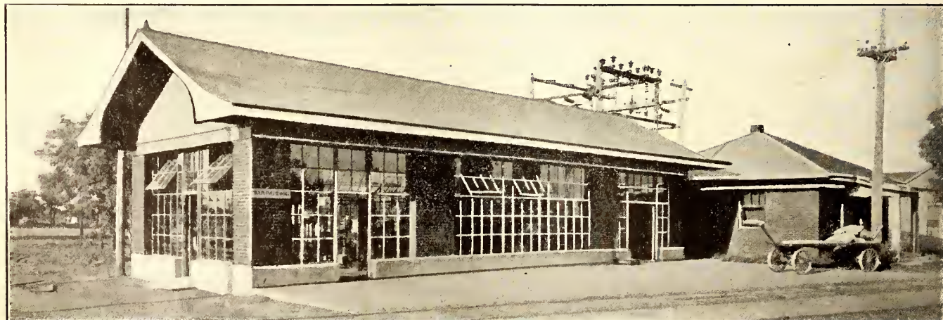
NEW KANSAS INTERURBAN—BURTON DAYLIGHT SUBSTATION
